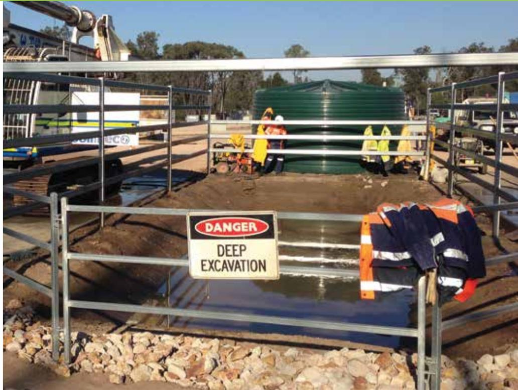
Biosecurity washdown facility established at the Wandoan TL construction yard – equipped with two washdown pads, a drainage sump, and a water filtration and recycling system.
