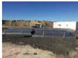
6 x Solar panels which connect to the container which houses the batteries.
